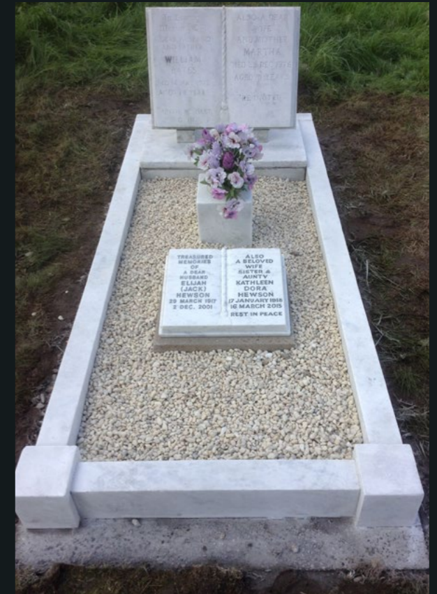
Completed restoration with addition of second book set and new chippings
